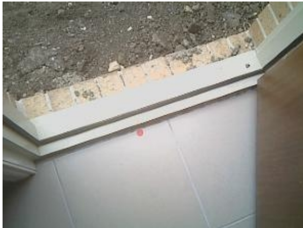
Tiles Tiling setout incorrect Minor Defect Type: F Tiling has been installed incorrectly, hence, a large grout joint has resulted that is not up to standard. Refer standard codes and tolerances document published by the Building Commission. Re-tiling should occur.
