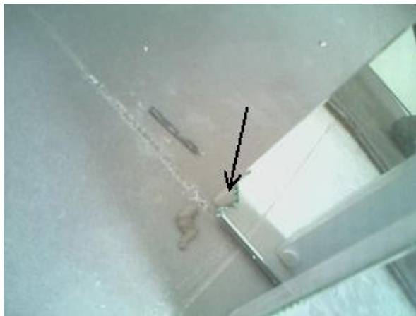
Built in robe/cupboard Damage glass to over head cupboard Minor Defect Type: A Requires replacement.
