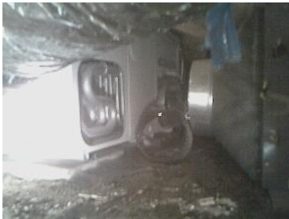
Air conditioning system Ducts not connected Require connection before commissioning.
