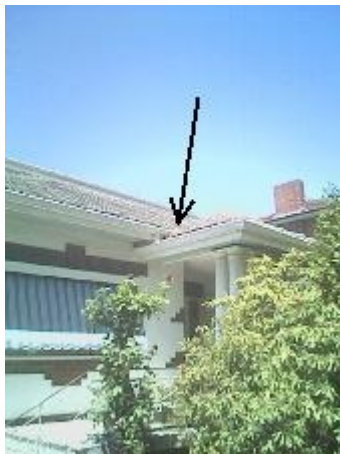
Valleys Corrosion in valleys Minor Defect Type: D Valley to the front elevation will require replacement in the near future.
