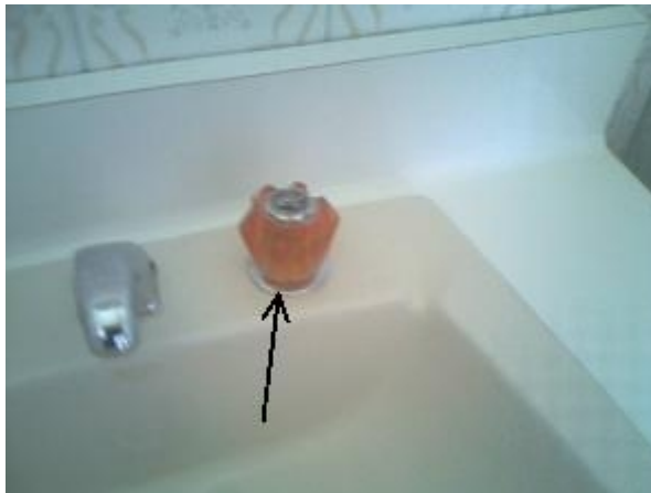
Wash basin taps Seized cold tap Minor Defect Type: A Further investigation required by a licensed plumber. Occurs to the bathroom on the 1st level.
